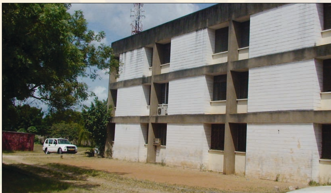
Figure 4.1: Existing Building in PPRA's Plot at Kurasini
