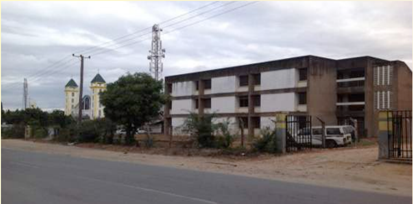
Photo 4-1: Existing building at PPRA plot in Kurasini, Dar es salaam
